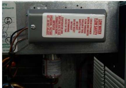
Generally the cause will be low or insufficient water flow caused by a clogged “Y” strainer or restricted flow in the process. This safety can also be tripped by low ambient conditions overnight or during shipping. Resetting this control and not determining the cause for tripping can cause the evaporator to freeze and rupture.
