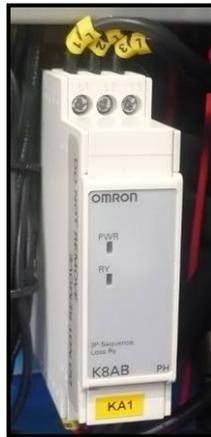
Phase Sequence Detector Relay inside the electrical box with the Power (PWR) and phase sequence (RY) indicator LEDs.
