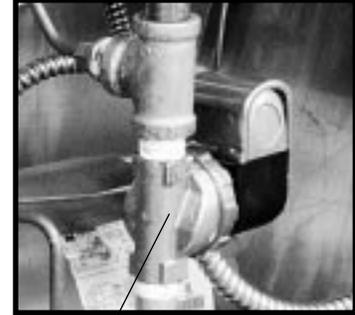
Typical cooling solenoid valve on RK units
